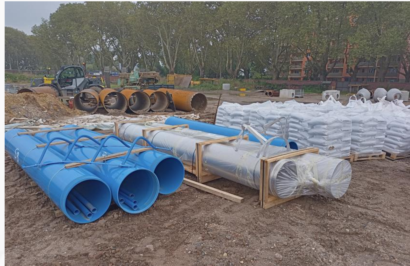
Brunnenrohre, Wickeldrahtfilter, Filterkies
